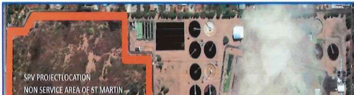
St Martin Wastewater Treatment Plant – SPV Project Location
